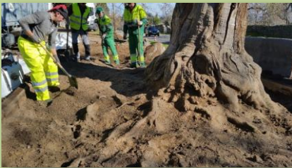
Addition of 8 m 3 of high quality topsoil
