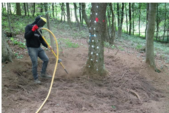
Fig. 128 Use of air excavation tool.
