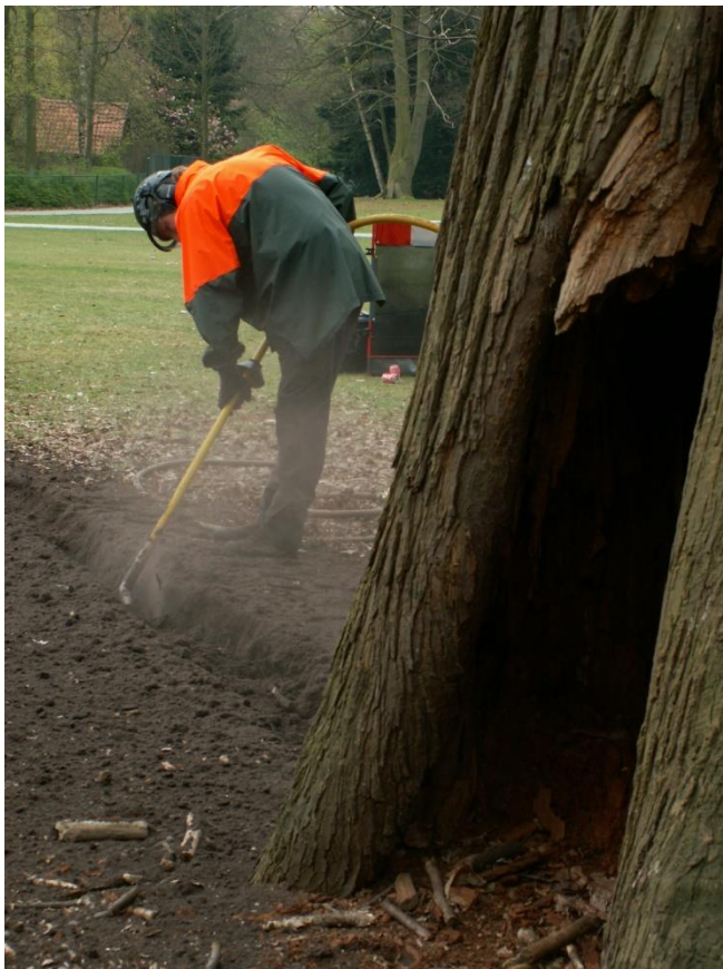
Fig. : pneumatic soil excavation around a veteran tree
